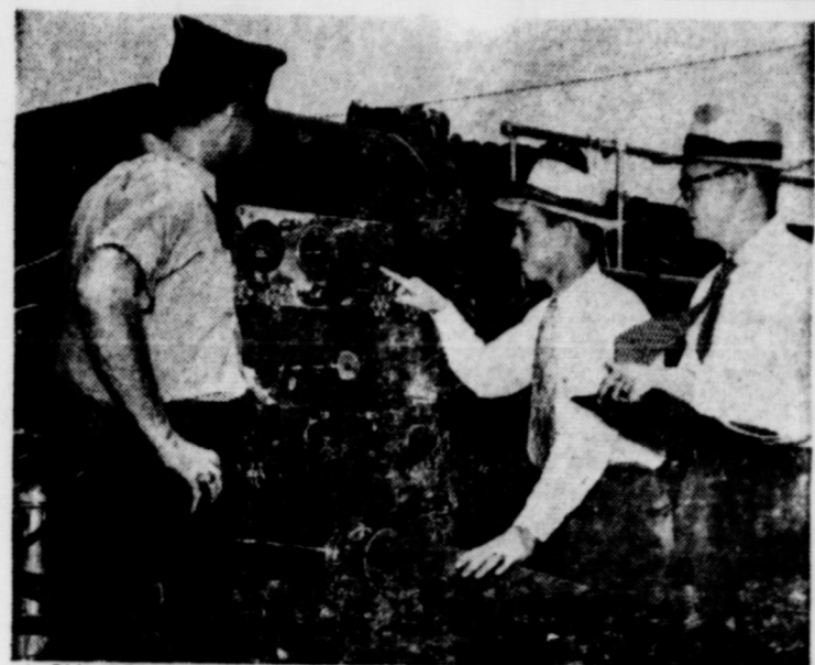
A PUMPER TRUCK isn't of much value to a fire department if it doesn't pump—and in sufficient quantity. Here a fireman watches while inspectors of the Fire Prevention and Engineering Bureau of Texas check a pumper's performance. Checking municipal fire defenses is just one of the many jobs performed by the Bureau as a public service of the fire insurance company.
