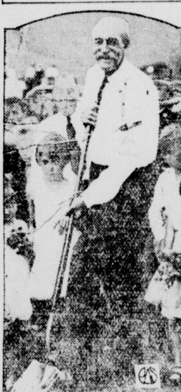
Governor Pinchot dug the first spadeful when work was begun on the Pymatuning dam, 25 miles above Sharon, Pa.
