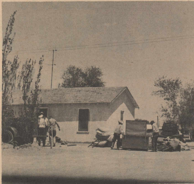
FIRE DAMAGE amounted to approximately $1200 to the home of A. C. Houston family. The kitchen suffered most of the loss while smoke damage was throughout the home. The Houston family is now making their home at the W. R. Reed's rent house.
