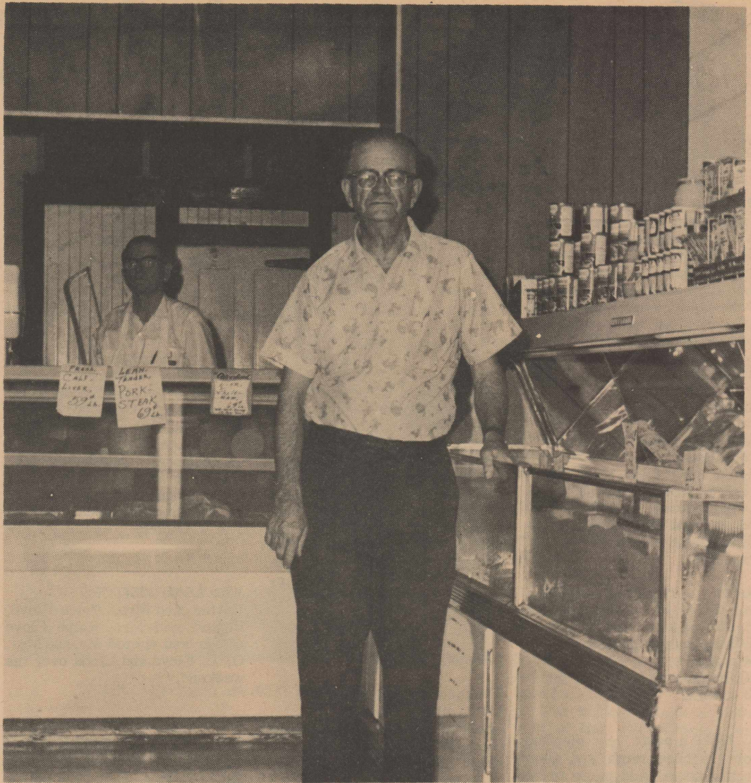
J.J. NEWSOM proudly stands before one of his many new refrigerator units which has been added to his newly remodeled store. His formal opening will be held Tuesday, Aug. 15 and Wednesday, Aug. 16. He and his son Stewart, will operate the home owned grocery.
