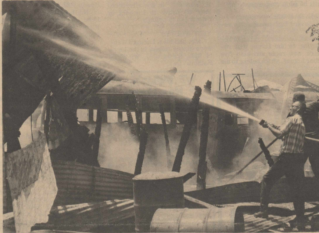
FIREMEN BATTLE BLAZE--Members of the Hart Volunteer Fire Department are shown fighting a fire that destroyed the Hart School bus barn and caused an estimated $5,000 in damage. In the background is a bus that was destroyed in the fire.
