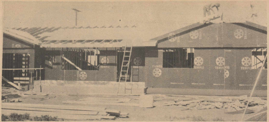
Under construction here is a new home for the Carl Rambos.
