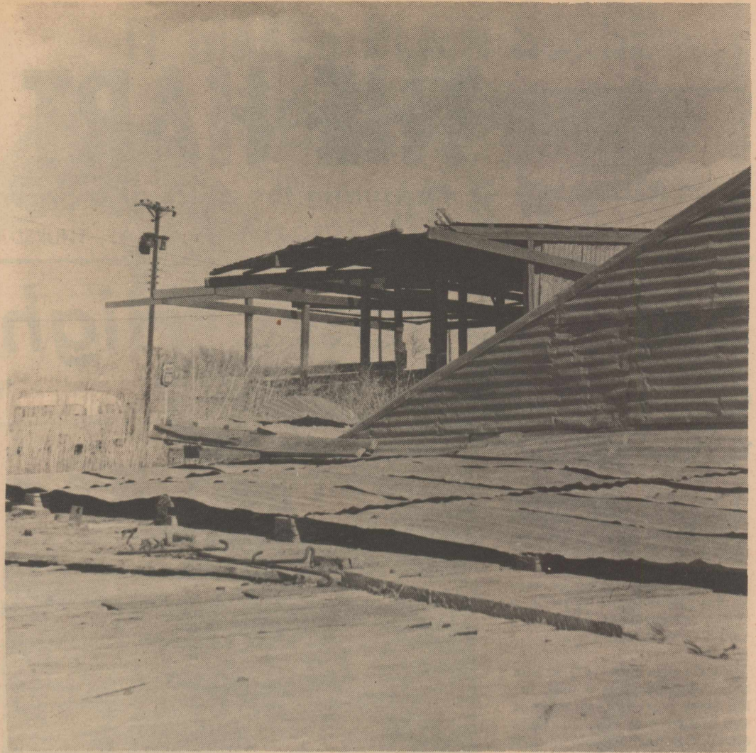
COLLAPSE CAUSED BY WINDS--The sides of the old potato shed in the south part of Hart were blown out by high winds last week, causing the roof to fall to the loading platform next to the railroad.
