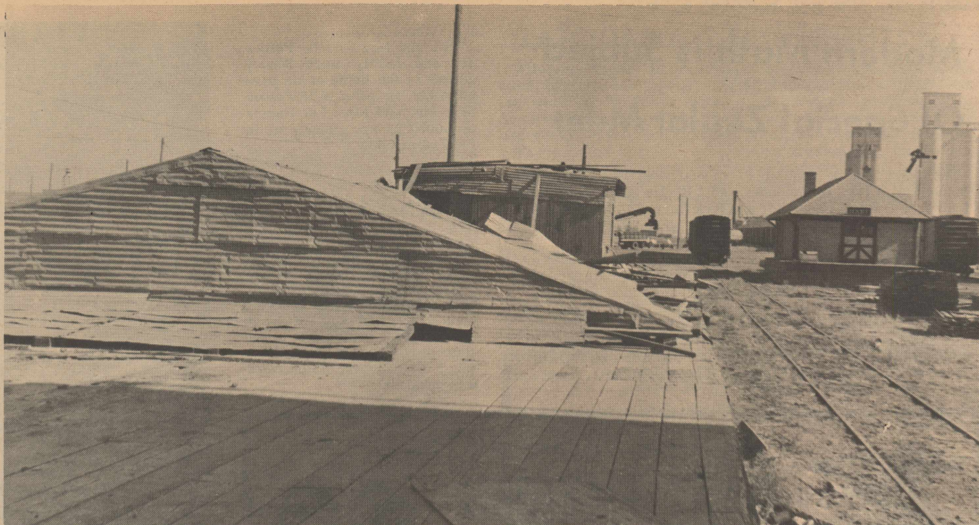
DESTRUCTIVE WINDS—High winds last week caused this old potato shed west of Hart depot to rip apart. Most of the shed which collapsed was made of tine sheets. It was not in use at the time.
