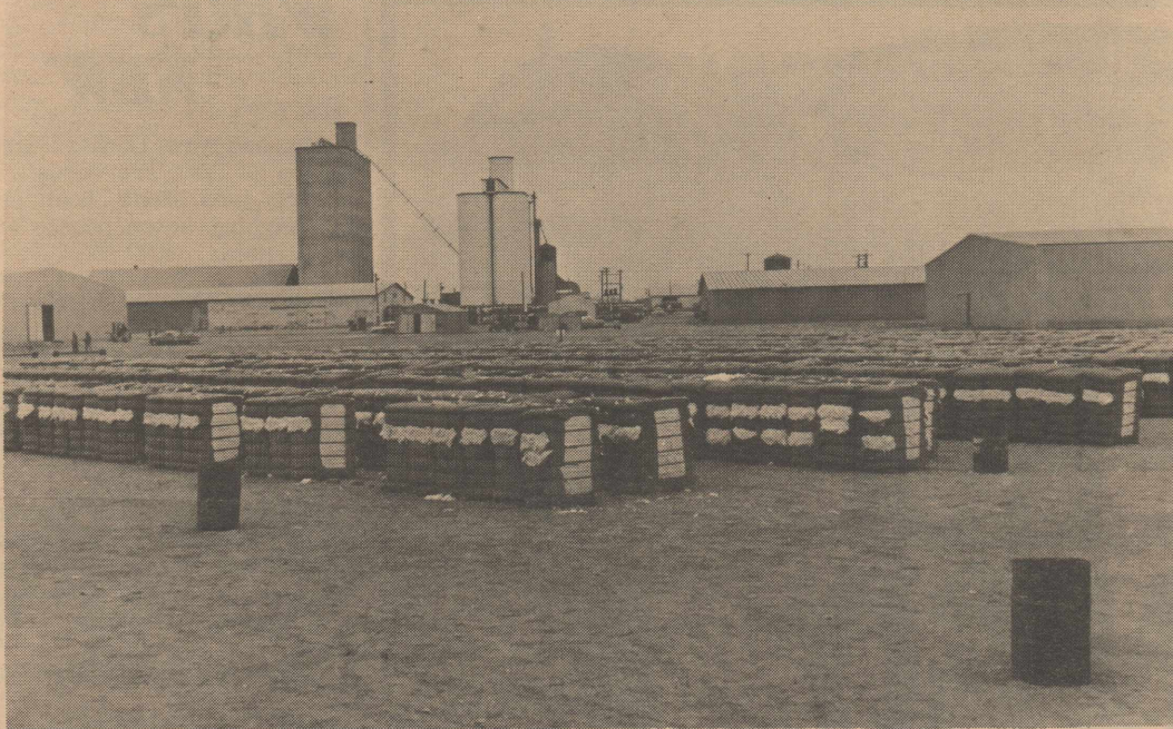
COTTON SEASON IN SWING--At least that was the case at Panhandle Compress in Hart Tuesday before the snow started, as workers rushed to ship out a near-record harvest. The compress serves seven area gins in Hart, Edmonson, Circle and Olton.
