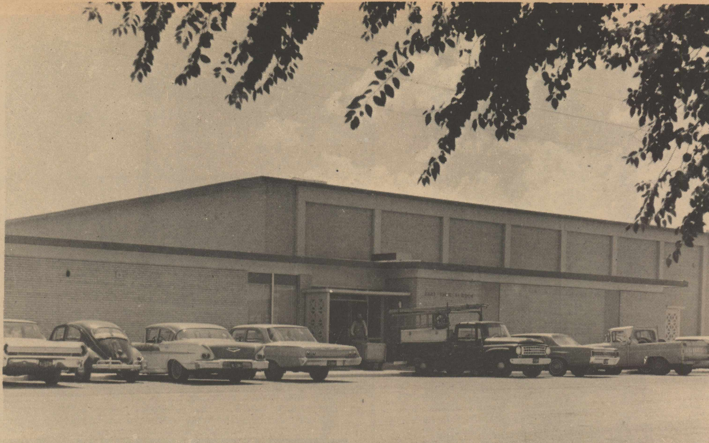
NEW SCHOOL --The new Hart Junior-Senior High School is right across the street from the old high school, as this picture taken from the front lawn of the old school should
