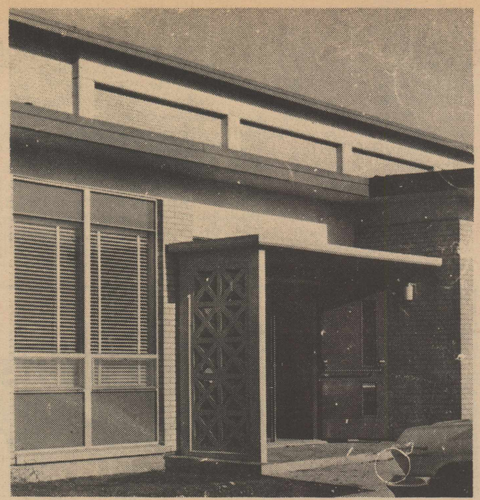
AFTER NEW SCHOOL --The new Hart Junior-Senior High School is compactly constructed, with only these two windows in the principal's office. The brick building and gymnasium is completely air-conditioned for year-round comfort.
