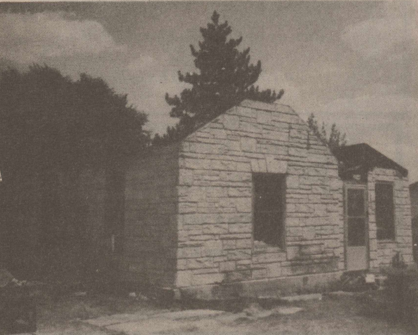
Jess and Deanna Mixon lost everything in the July 4th housefire. Wiring overload was believed to be the reason. The fire had burned for approximately one to one and a half hours before reported. It started in the Northeast corner bedroom.
