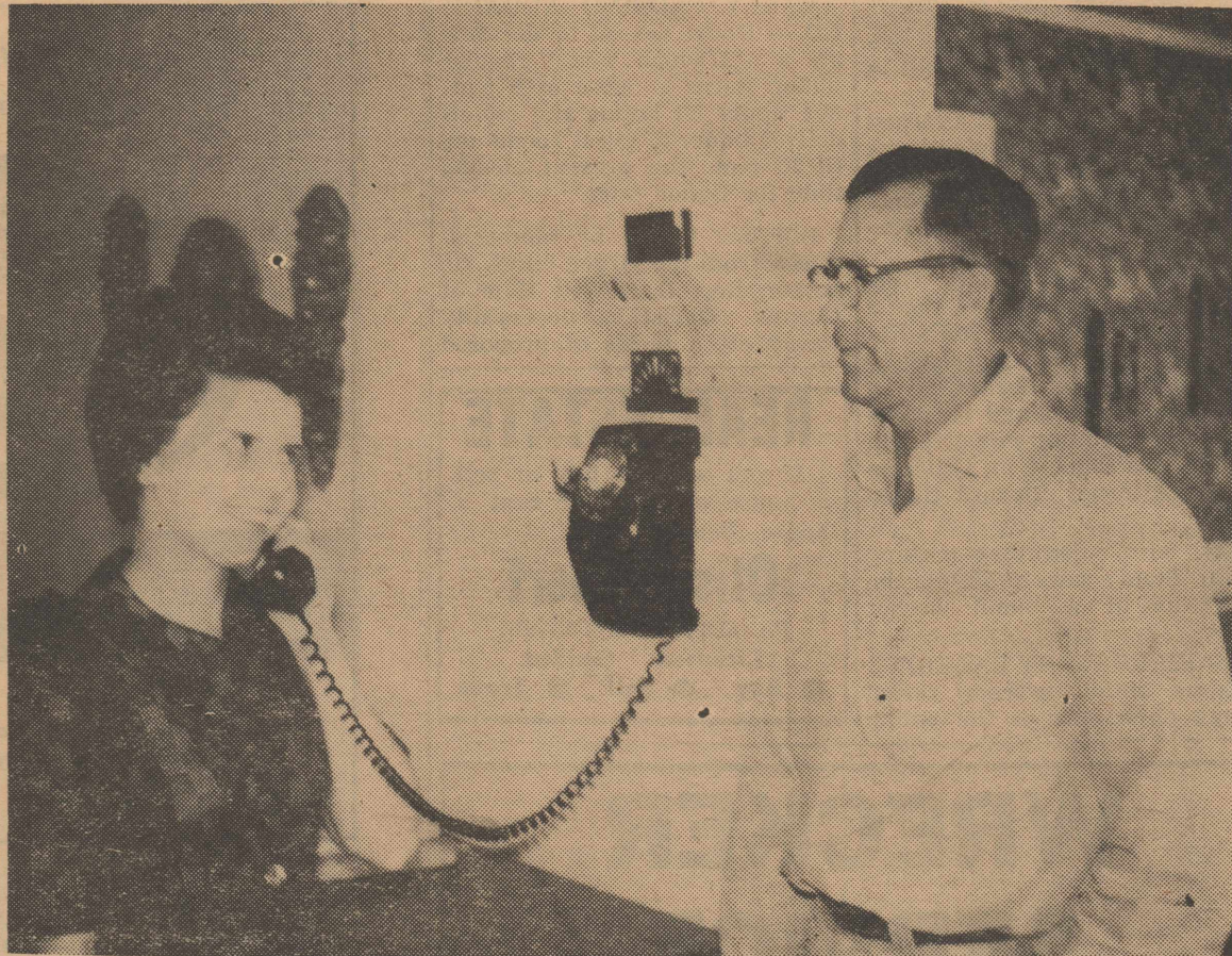
HAPPY GENERAL SUBSCRIBER — Mrs. Wyndoll Stephens is shown above admiring the new telephone General Telephone Serviceman Bill Smith has installed. Another representative of the company, Jack Shelley, of Seymour, commercial representative, was also on hand to give Mr. and Mrs. Stephens a desk set for being the 1,000th telephone subscriber in Knox City. There are 1,007 telephones in use here today, and the company, in keeping abreast of the situation has already added 100 new phones to this office.
