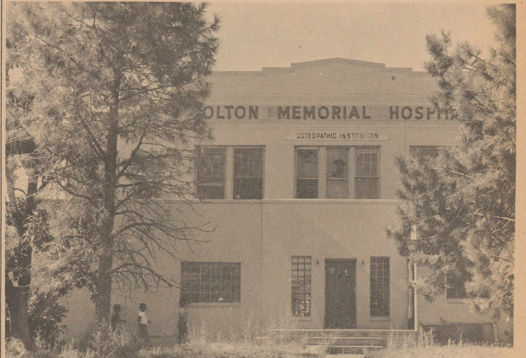
ONE LAST LOOK —Olton Memorial Hospital is shown as it looked last week, right after workers began razing the interior of the building. A demolition crew will pull one wall of the structure down this weekend, and the rest of the building will be demolished during the next two weeks.
