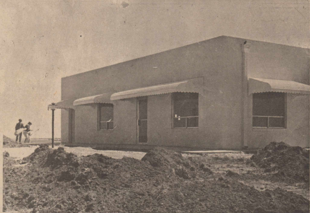
JOB COMPLETED - Here is an outside view of the new community building at Olton Recreation Center. The building has been completed and an open house is scheduled April 30. New awnings put on this week added an extra touch to the structure.
