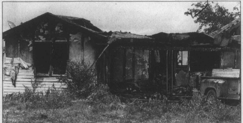
House destroyed ... This house, located just north of the TxDOT facility on the US 87 access road in Tahoka and reportedly vacant, was destroyed in a fire about 1 a.m. Oct. 8. The State Fire Marshal is investigating the fire. (LCN PHOTO by Juanell Jones)
