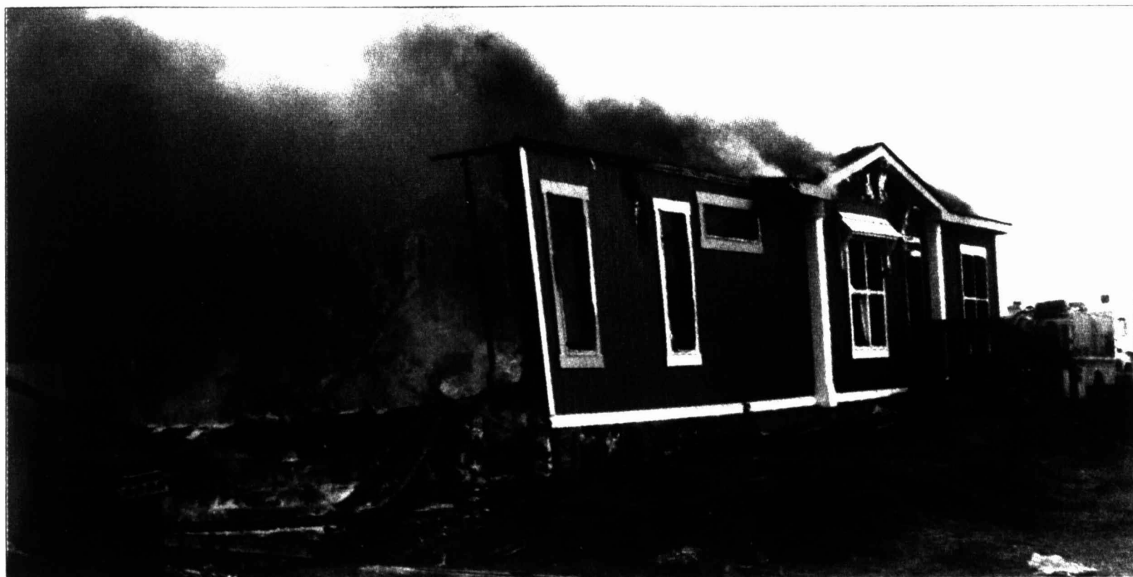
Family loses home ... The family of Dr. Charlie Snider lost their home in a fire last Wednesday afternoon, with New Home Volunteer Fire Department responding at 1:53 p.m. to 1177 CR 6, just north of New Home. The blaze consumed the mobile home and all its contents, but fortunately no one was inside the home at the time. According to a facebook post, a GoFundMe account has been set up for the Snider family to help with expenses, as he and his wife and young child reportedly lost everything except for the clothes they were wearing at the time of the fire. Their horses, in a nearby barn, were reportedly okay. (LCN PHOTO by Gary Jones)
