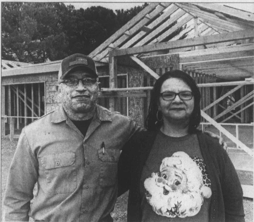
Hometown project ... Tahoka's Raymond and Janet Lara have more than a decade of renovating older homes into beautiful properties here, and are now involved in their first new construction project — two duplex units on North 5th Street.
