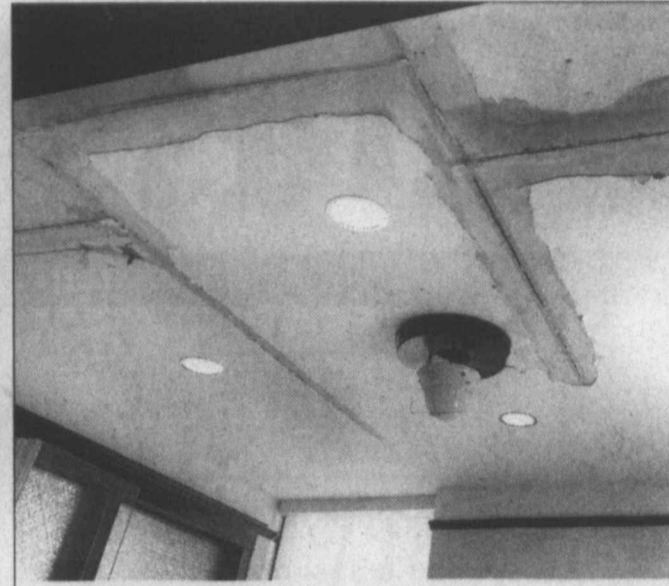
Courthouse ceilings ... Many of the ceilings in the lower three levels of the Lynn County Courthouse are cracked and peeling plaster or sheetrock, after the recent flooding mishap at the courthouse. County Judge Mike Braddock said it is estimate at $100,000-$150,000 just to repair sheetrock and plaster issues, and damage assessments are still underway. (LCN PHOTOS by Juanell Jones)
