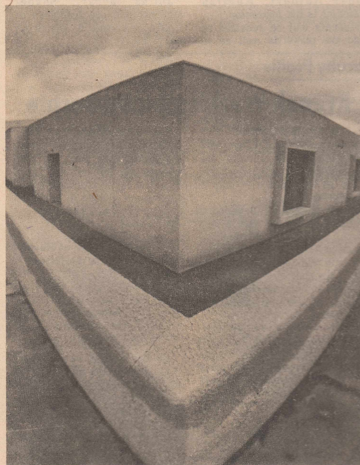
WHAT IS IT? — Some say Noah's Ark has washed ashore at WTC, but actually this is a photo of the Academic Science B building, taken from a unique point of view. (photo by Jim Severs)
