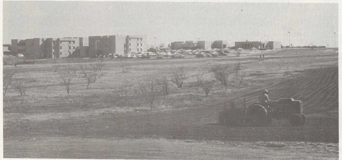
GOLF COURSE PROGRESS — Maintenance crews continue construction in the campus pro shop (above), while work on the fairways resumes after recent cold, wet weather. (photos by Debbie Sutton)
