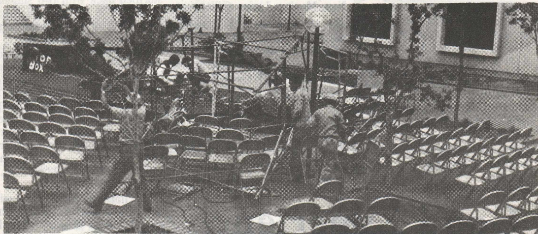
The maintenance crew gave their time and effort to help put the Sentell Memorial Stage back in condition after the windstorm.
