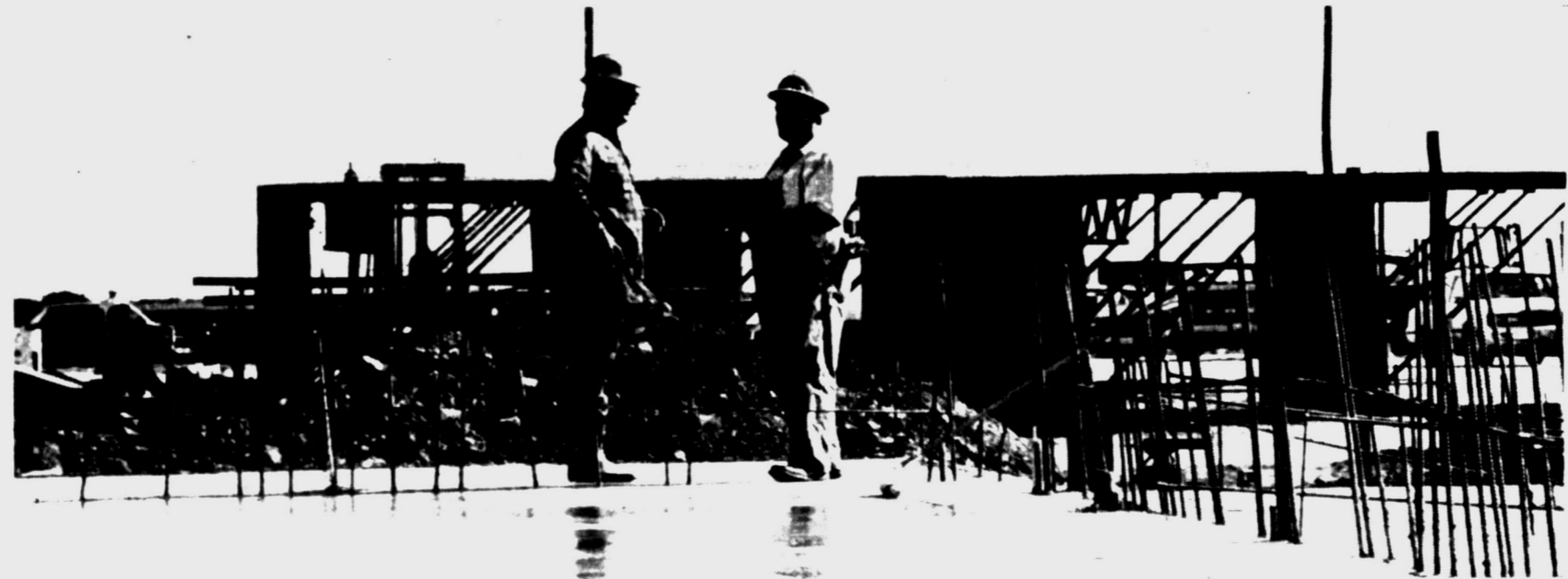
PRISON SITE — Some 80 workers are now at the site for the Texas Department of Corrections prison here with the number expected to expand to 200 by December. Officials say the work is now approx-
