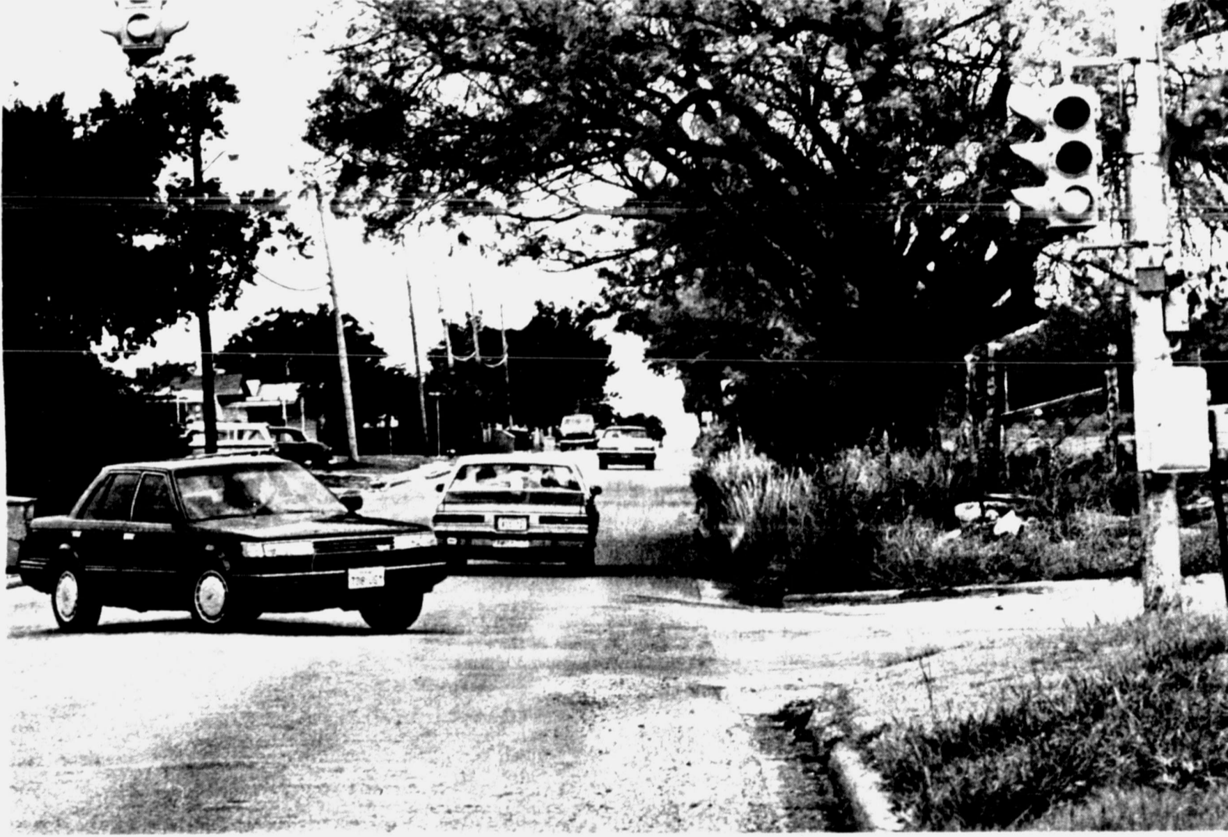
WIDENING PROPOSED — This section of 37th St. looking west would be widened some 6 ft. on the north side (shown at right) and some 4 ft. on the south if plans are approved to widen the city roadway west from College Ave. to Crockett Ave. This photo was taken at the intersection of Ave. V. Plans are to make 37th a four-lane rather than two-lane traffic route along this .6 of-a-mile stretch. (SDN Staff Photo)
