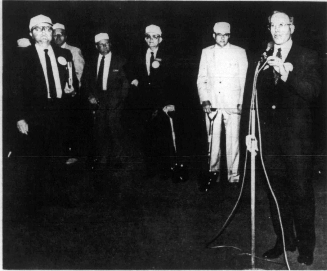
GROUND BREAKING — At Monday's ground breaking, TDC Board Chairman Charles Terrell of Dallas (right) was complimentary of the Scurry County bid package put together to secure a 1,000-man TDC unit here. Terrell commented, "Of all the towns and cities that sought state prisons, I
