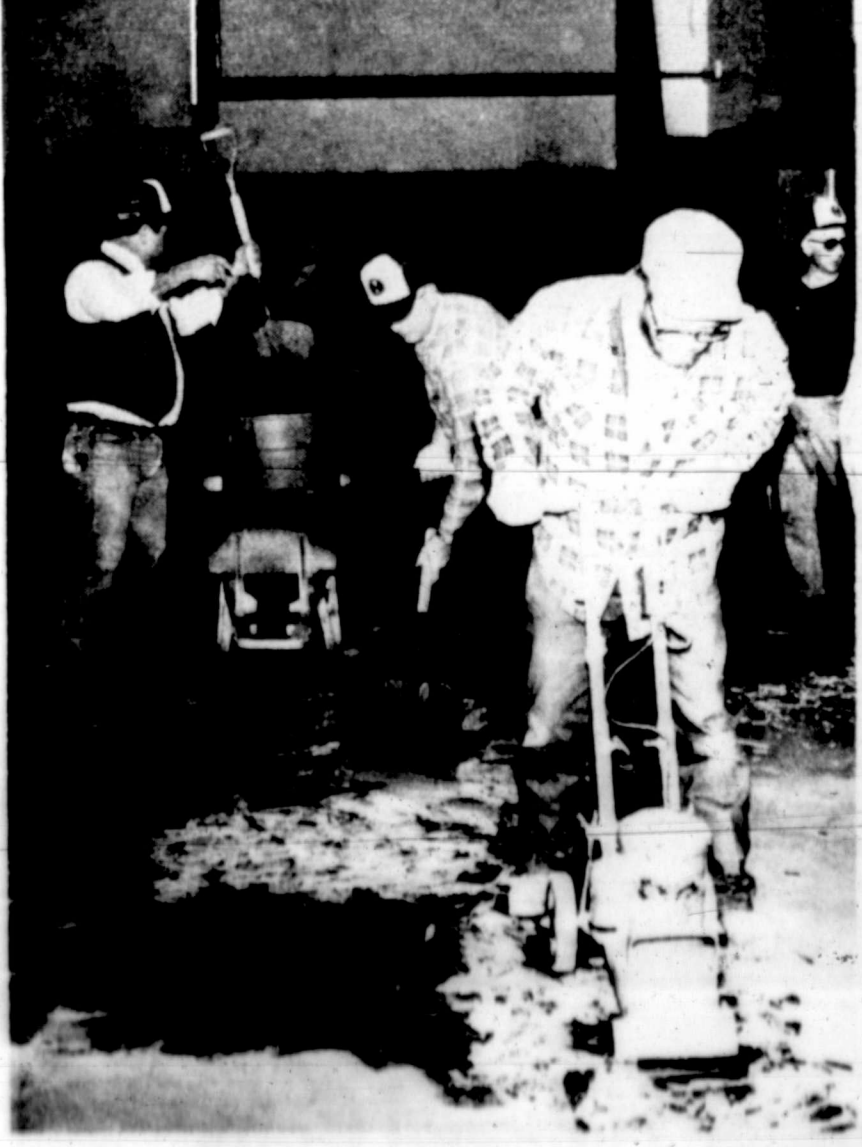
GETTING IT DONE — Vietnam veterans and American Legion members got a fast start in tearing up the old tiles in the Boys Club gymnasium Thursday night. The groups have already raised enough money to have the floor re-tiled. (SDN Staff Photo)
