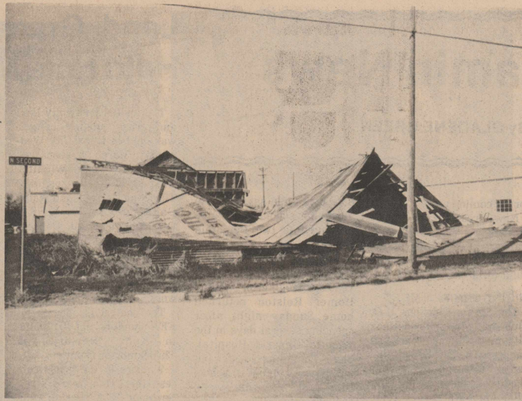
NIGHT CAME Early Tuesday of last week when a dust storm roared into town, painted the sky a dark orange, and reduced visibility that cars used their headlights. The above tin building belonging to a long ago firm, Porter and White, at the corner of North Second and Aspen, could not withstand the gusty winds which were clocked on the Cable 2 Scanner up to 80 miles per hour.
