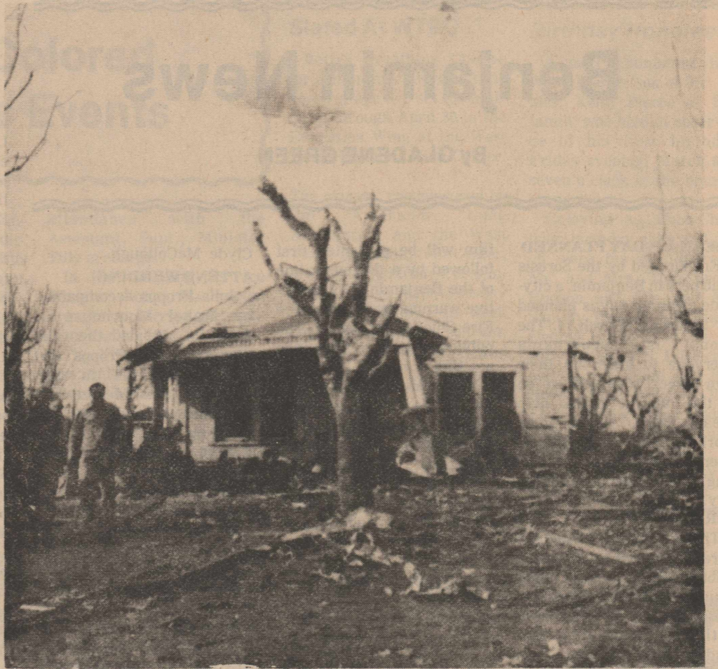
BADLY DAMAGED was this home belonging to the late Mr. and Mrs. Benton Anderson at the corner of South Fourth and Avenue G. The house was later remodeled and is now occupied by Daniel and Christene Greene.
