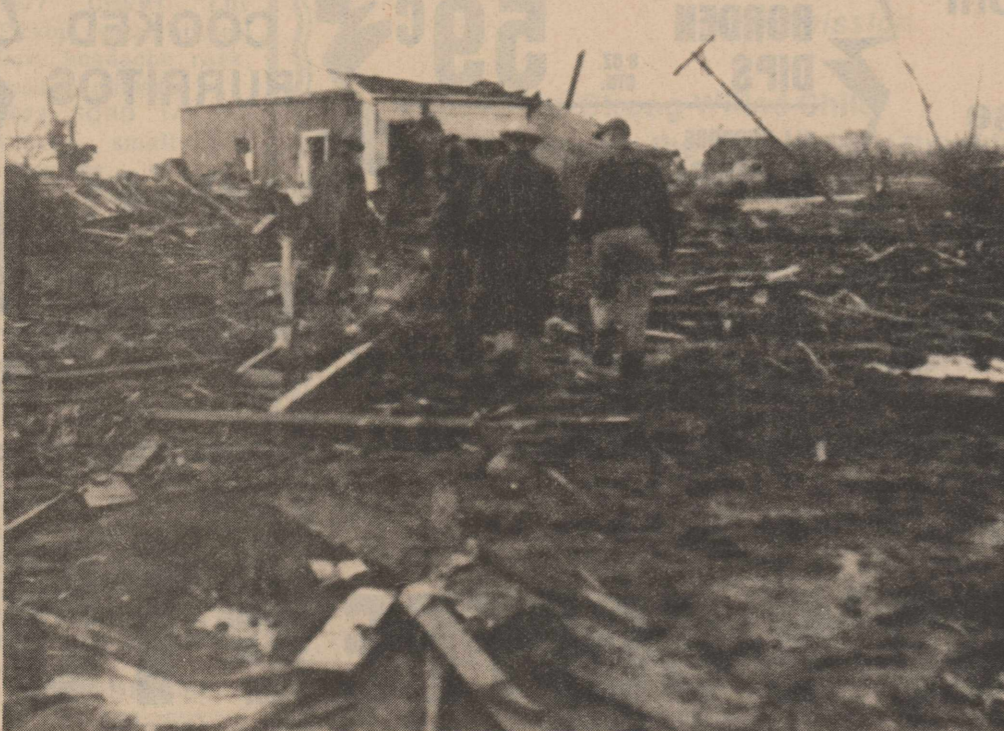
IN PATH OF DESTRUCTION
