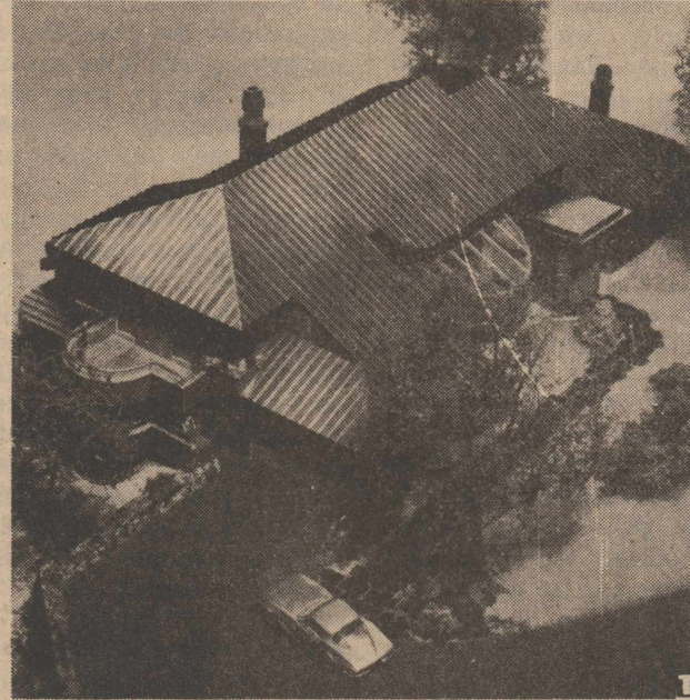
Under the dramatically sloping copper roof of this elegant model solar home near Stamford, Conn., are highly advanced computers that can do everything for the family from controlling the home's various solar heating systems to recalling what was served at past dinner parties and who attended.
