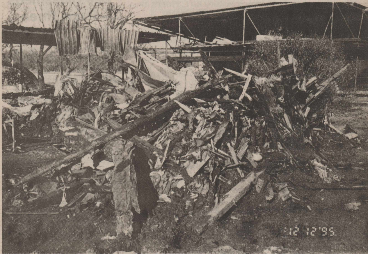
A BURNED PILE OF RUBBLE is all that remains of the Acevedo home in Benjamin after a fire last Friday afternoon that destroyed everything belonging to the family of two adults and nine children. There were no injuries in the fire, but the family was left with just what clothes they were wearing when the fire engulfed their wood frame home. (NEWS Photo)
