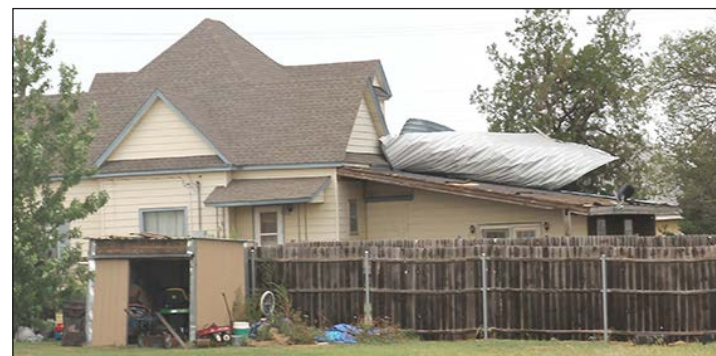
A portion of the roof of the Larry Kidd house was peeled away by the wind. ENTERPRISE PHOTO / ROGER ESTLACK
