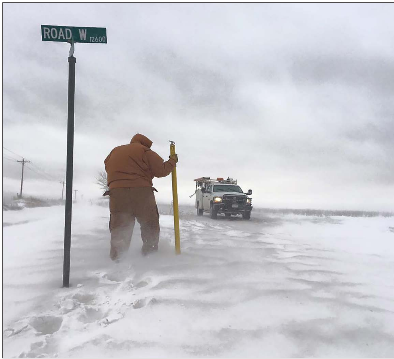
Greenbelt Electric lineman Levi Proaps trudges back to his truck through blowing snow after repairing a service at the intersections of County Roads W and 14 southeast of Clarendon last week.
