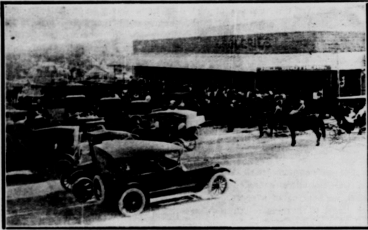
A STREET SERVICE IN LOMETA
