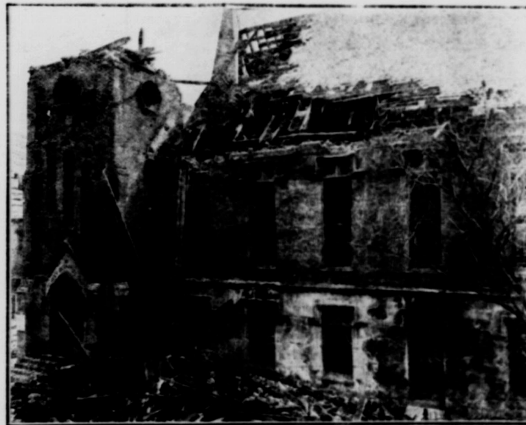
HISTORIC FELICITY STREET CHURCH WRECKED.
