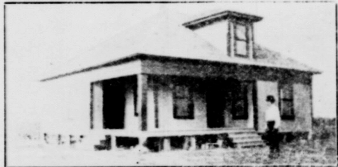
PARSONAGE AT LAKE CREEK, TEXAS.
