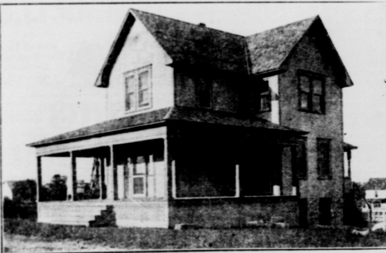
METHODIST PARSONAGE, BLANKET, TEXAS.
