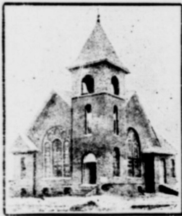
BOULEVARD METHODIST CHURCH, Fort Worth, Texas.
