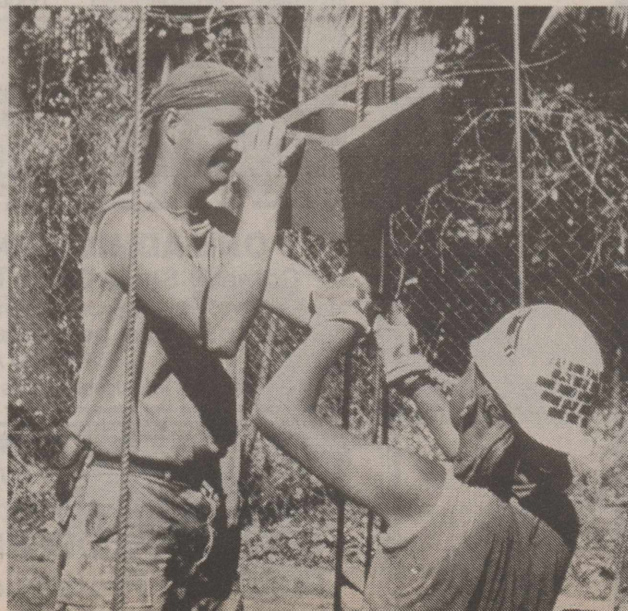
A1C Chris Watson lowers a cement block to SSgt. Daniel Carrington during the 64th CES Prime Beef deployment to El Salvador. The men were helping erect the exterior wall to a new school building. At far right, MSgt. Robert Stalker runs a compactor over the ground at one of the two school construction sites.
