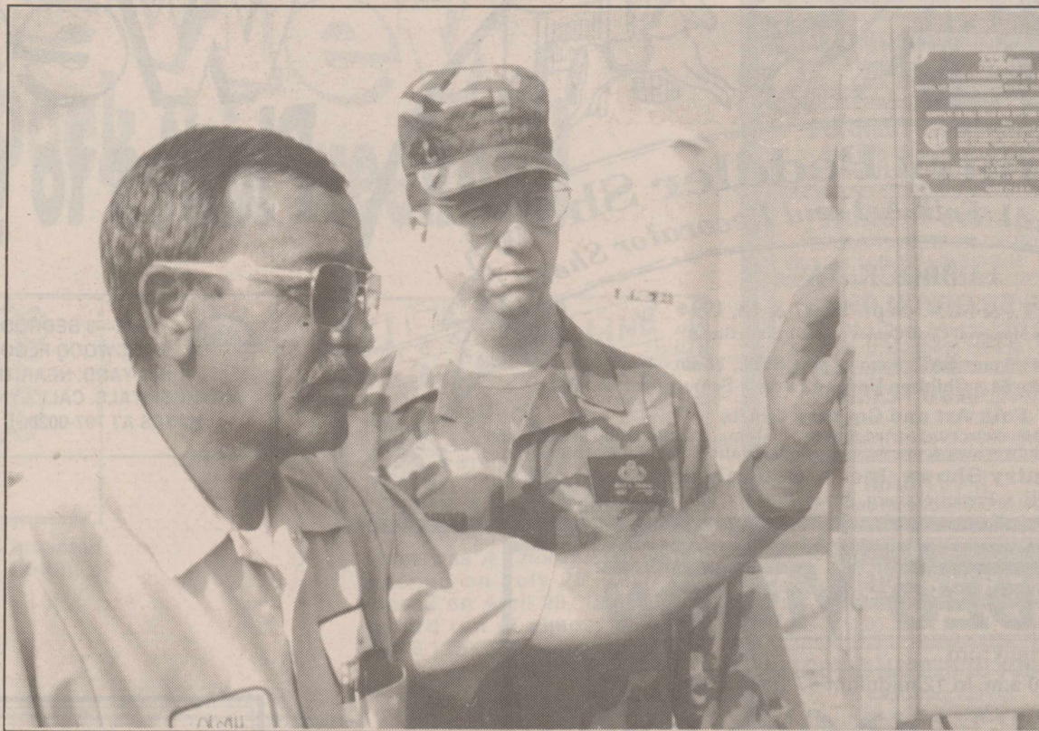
Mehmet Olcay, a contract fuels storage attendant, checks one of Reese's jet fuel storage tanks as MSgt. Kelly Starbuck 64th Logistics Squadron, monitors the operation of the new high-tech equipment. At right, Olcay shows how attendants had to scale the tanks to obtain measurements before the arrival of the new equipment.
