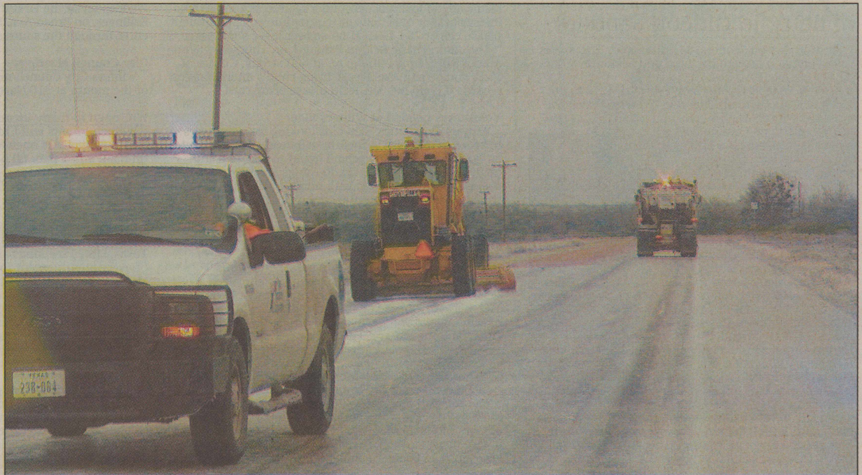
A thick sheet of ice covers Hwy 158, north of Ballinger, as Texas Department of Transportation crews work on making the roads safer by dropping sand and removing the ice.
