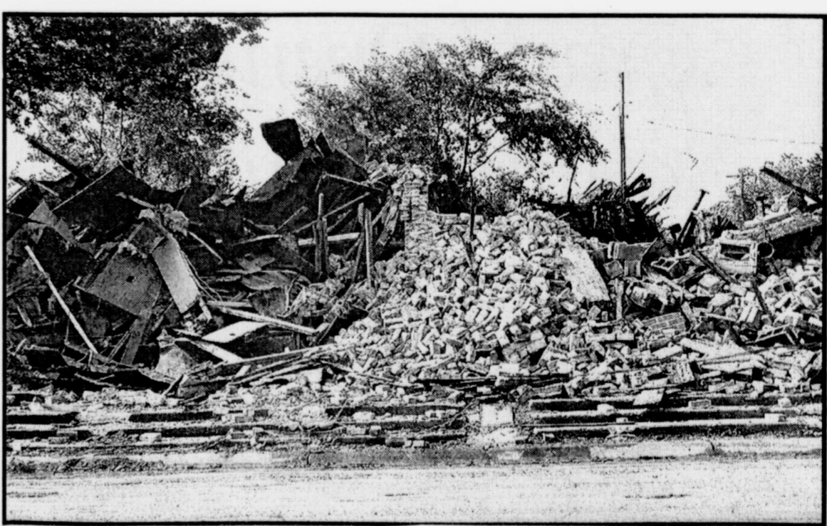
DESTROYED BY FIRE-the old Masonic Lodge Building in Talco was destroyed by fire last week. The building which was built in the mid 1930's once housed not only the Masonic Lodge and Easter Star groups but below at one time Westbrooks Grocery and other businesses. In recent years the lower floor has been apartments. The main street in Talco has lost yet another of its historic buildings. (Staff Photo Nancy Brown)
