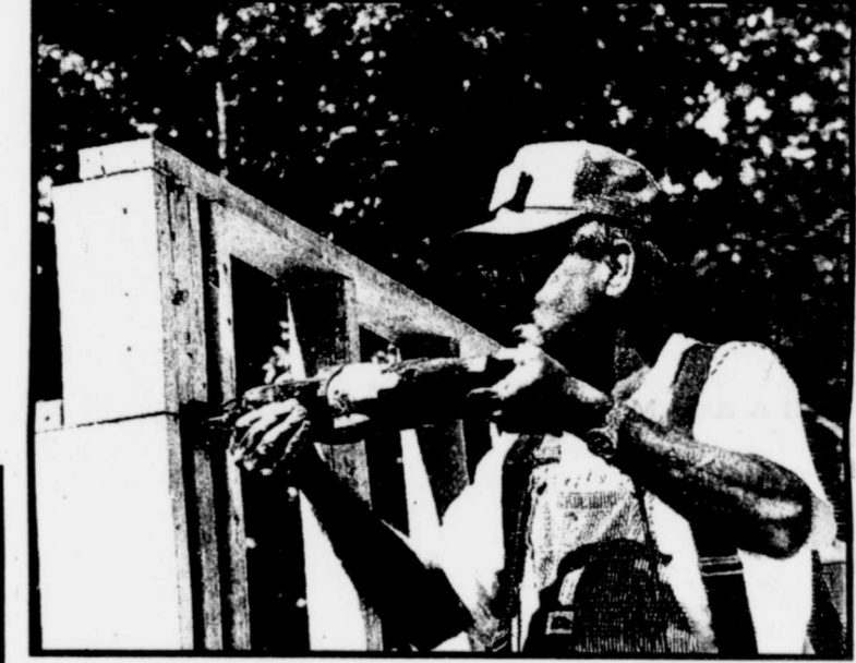
EDDY DENNY , member of the First Baptist Church of Bogata, works on a Texas Baptist Men Retiree Builders construction project near Paris, building a home for an 11 year old girl and her family.
