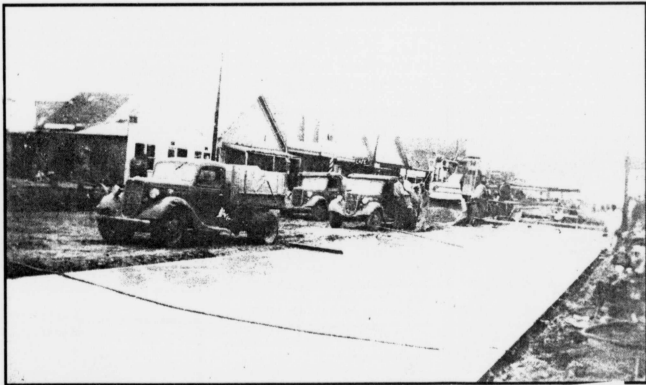
ROAD PAVING-This photo sent to the Talco Historical Society shows the first paved roads being put down in Talco following the oil boom. Construction workers how would you like to use this equipment today? For the era it was the best!
