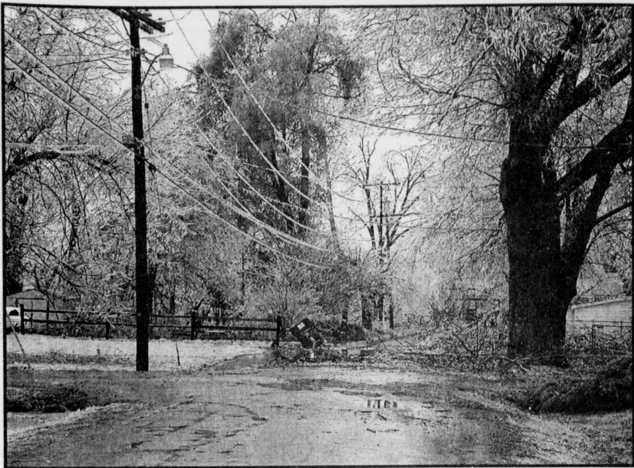
ICY POWER LINES-these power lines, lowered by ice and beset by fallen limbs, are an example of some of the problems the power companies have had to face since the worst ice storm in memory devastated the area last week. (Staff Photo by Thomas Nichols)
