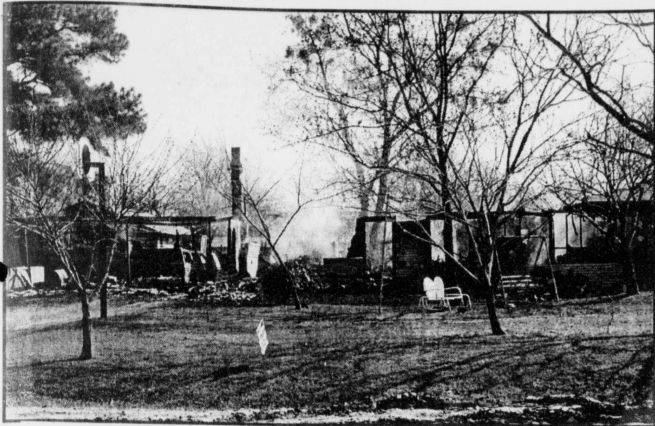
DESTROYED -The home of Mark and Jana Hawkins and children in Johntown was destroyed by fire late Sunday night and early Monday morning. Jana and youngest daughter, Hana, were the only ones at home when the blaze broke out. The two escaped with their lives but nothing was saved from the burning home. The cause of the fire was unsure at press time. (Staff Photo Nancy Brown)
