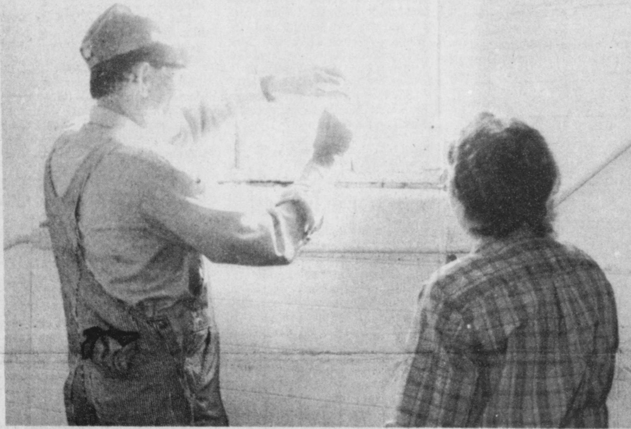
CLEAN UP -The Talco School was broken into, and workers were busy this week replacing
