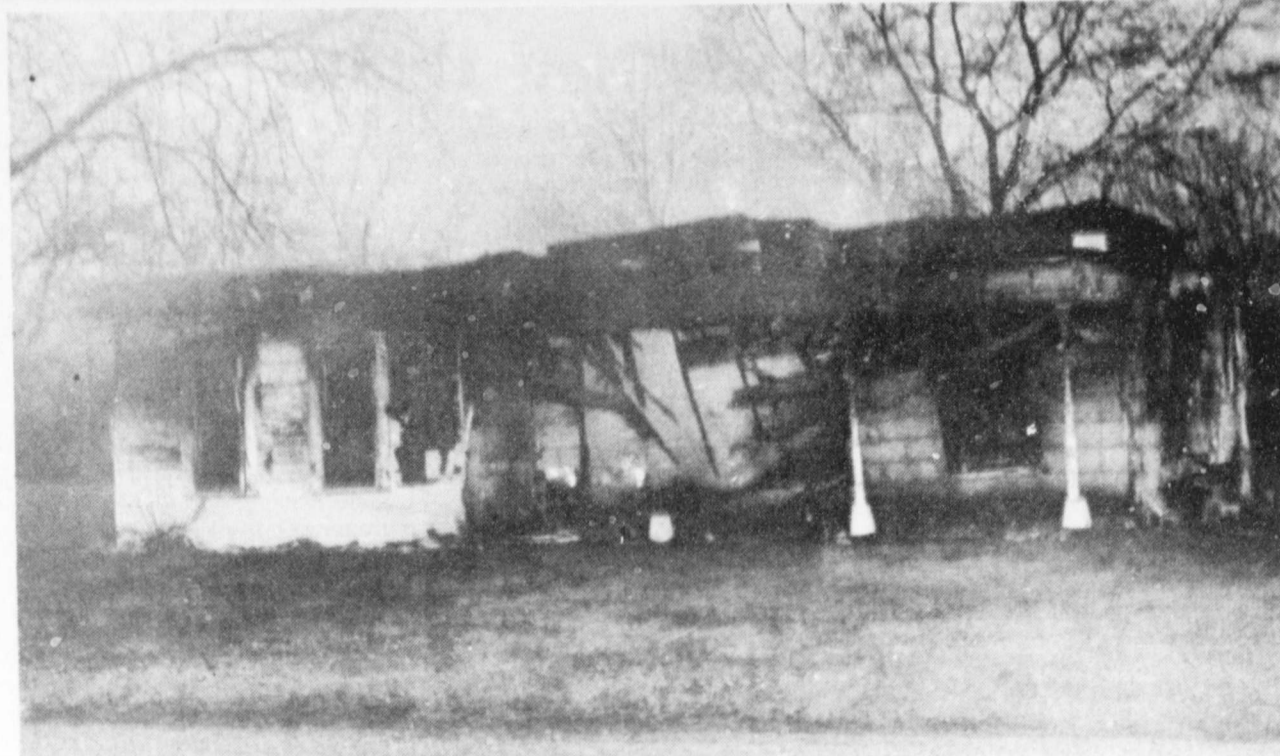
FIRE DESTROYED this home on Sixth Street in Talco Sunday night. The house was being occupied by Lary Kersey, who wasn't home at the time. Fire Chief Randy Carroll was injured at the scene. (Staff Photo by Jelu Binion)
