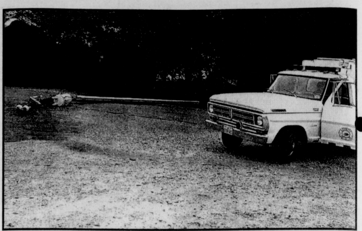
EARLY WEDNESDAY MORNING, a utility pole with a transformer crashed to the ground, closing the street east of Pattonville Auto and Truck Repair. Ed Ring, owner of the business, stated he heard a cracking noise and looked at the sound just in time to see the pole fall. The street was closed to through traffic for most of the morning while Texas-New Mexico Power Company made repairs and set a new pole. Businesses on the north side of U.S. 271 were without electric power while repairs were made.
