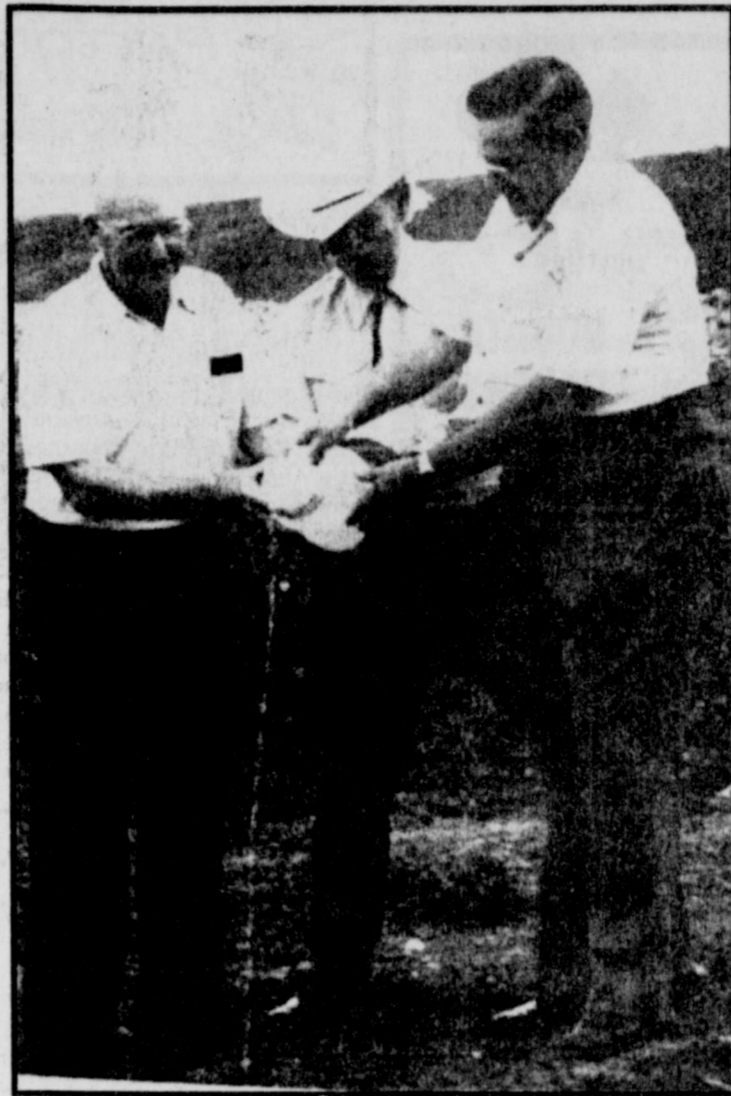
LONG AGO -in September of 1980 Albert Roach, left, Hugh Jeffus, Sr., and Deport Mayor Charles Foster poured the first "official" gallon of water into the newly built Tom Jeffus Water retention Structure. (Staff Photo by Nanalee Nichols)
