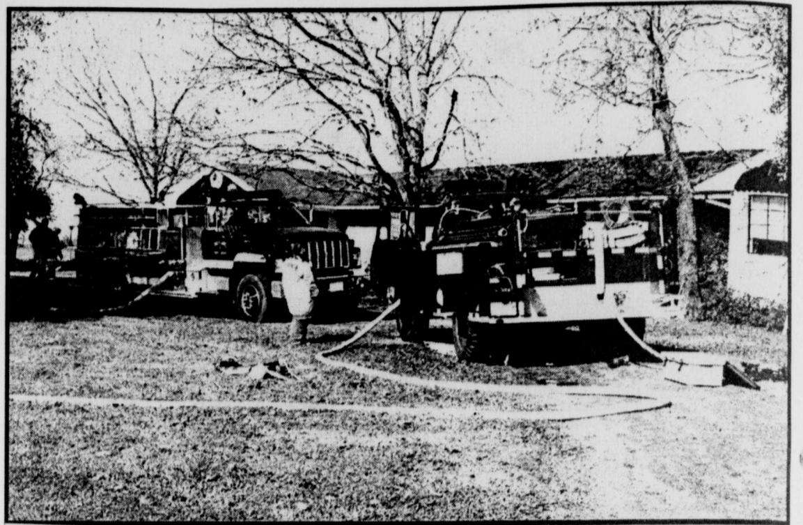
THE HOME OF Carol Dorsey, 718 Monroe St. in Deport, was extensively damaged by fire last Friday. Firefighters from Deport and Pattonville battled the blaze for over two hours. According to Deport Fire Marshal Thomas Nichols the fire was electrical in nature and originated in the kitchen. (Staff Photo by Thomas Nichols)
