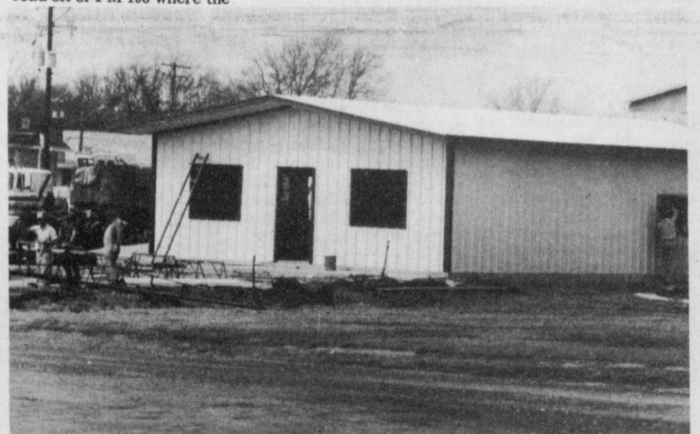
DEPORT FARM Supply is in the dry and further construction continues.
