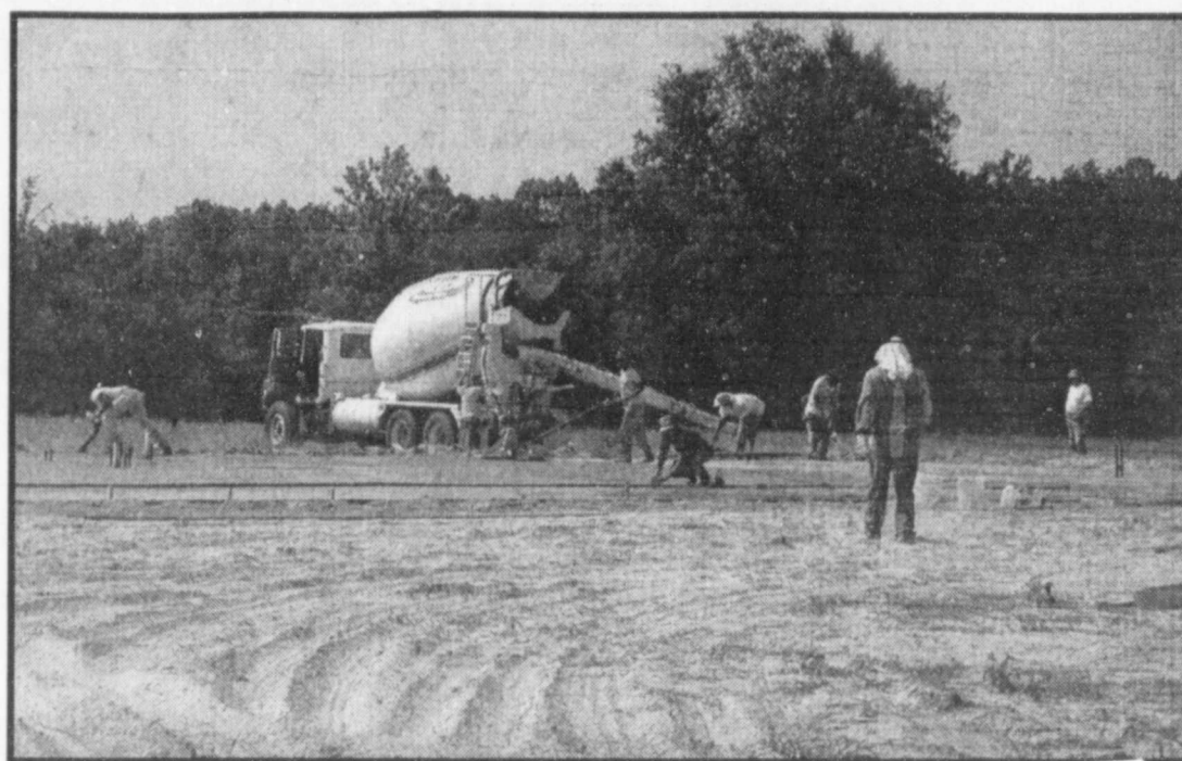
NEW BUS BARN AND ISS/AEP CLASS ROOM-Workmen were busy Tuesday pouring concrete for the new bus barn and ISS/AEP class room. The new facility will be a great improvement for those students who are unfortunate enough to make use of them and the new bus barn will be a very nice move for Transportation Director, Ricky Kennedy and staff. (Staff Photo Nancy Brown)
