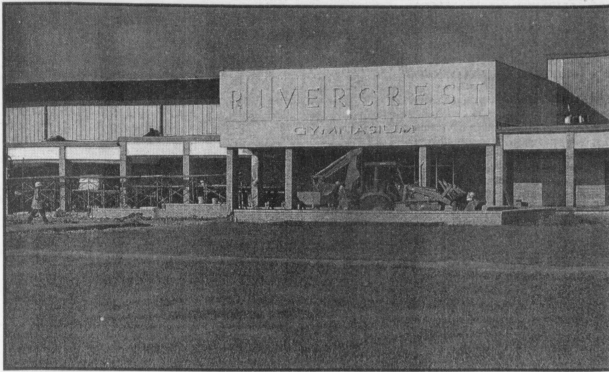
REBEL GYM will be ready by the time basketball season arrives according to contractors. The new structure will be a source of pride for coaches, students and members of the communities. (Staff Photo Nancy Brown)
