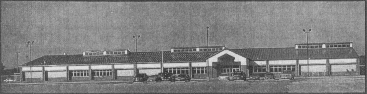
ALMOST READY -Teachers and staff of the Rivercrest School District were busy this week moving into the new elementary school located on Hwy. 271 near Rivercrest High School. The school will hold an official open house soon. (Staff Photo Nancy Brown)
